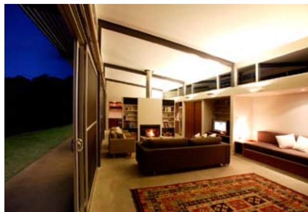
Interior of residence with good cross ventilation, thermal mass in an exposed concrete slab floor, and low VOC (volatile organic compounds) finishes
