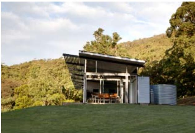
Kangaroo Valley house with shading devices to north glazing, water tanks and flowing indoor-outdoor space.
