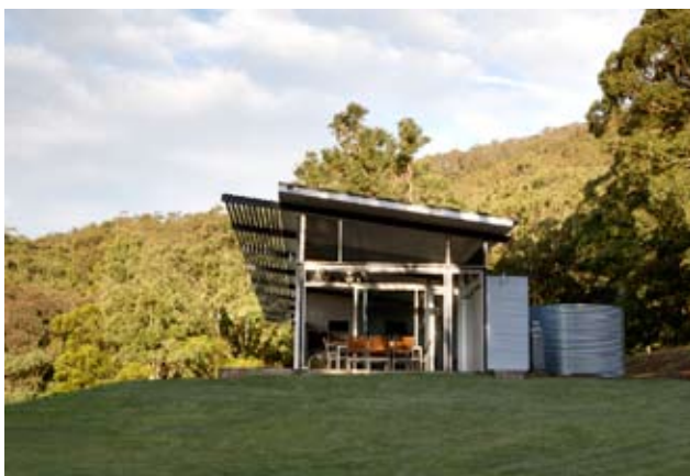
Kangaroo Valley house with shading devices to north glazing, water tanks and flowing indoor-outdoor space.
